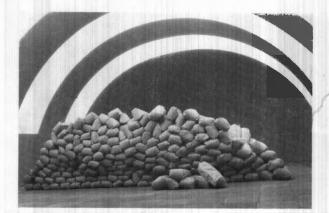
These halls are held up entirely by inflated air. Suitable for indoor tennis courts, warehousing premises, building construction carried on in all weathers under cover, and various other uses.
